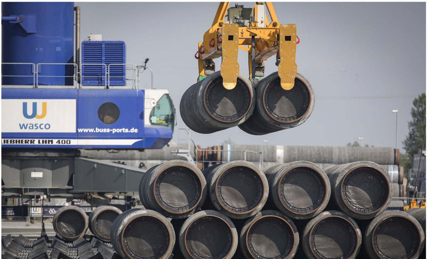
A crane moves Nord Stream 2 pipes at the Mukran port June 5, 2019 near Sassnitz, Germany | Axel Schmidt/Getty Images
