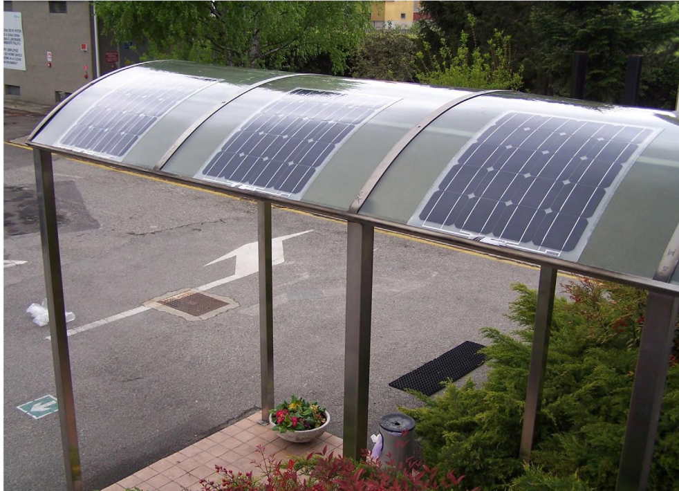
SABIC launches first polycarbonate building-integrated photovoltaic panels for roofing, cladding, and glazing applications.
