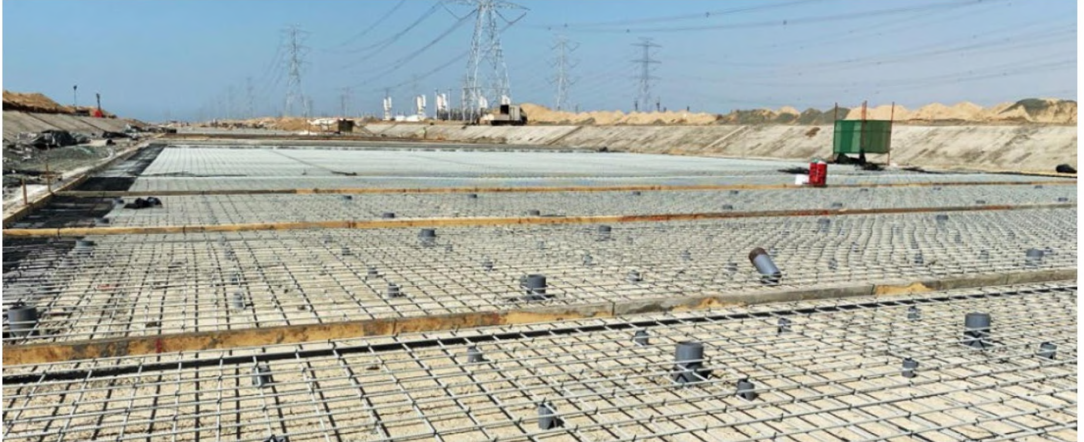
Jazan Flood Mitigation Channel
