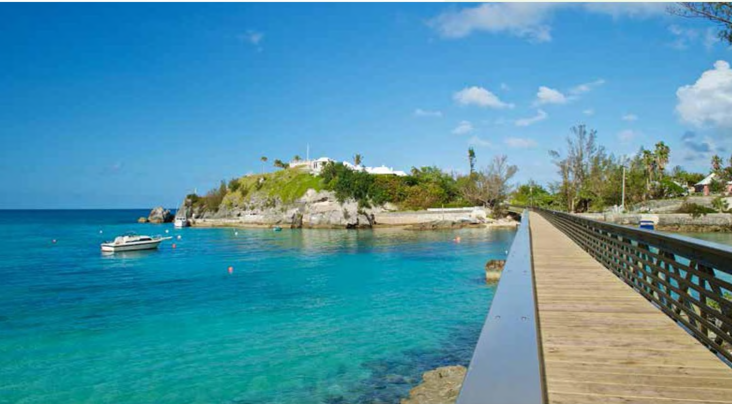
Bailey's Bay footbridge
