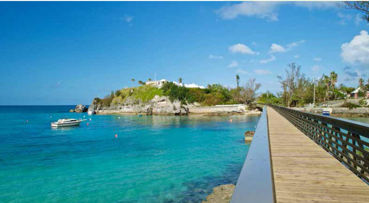
Bailey's Bay footbridge
