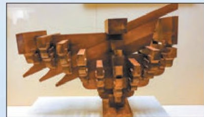
Center: The Hall of Supreme Harmony of the Forbidden City is a prime example of the traditional timber-framed structures that have withstood the test of time. Left top: The roof of the hall is decorated with figurines at the end of its diagonal ridges. Left: A model of dougong (interlocking brackets) on display at the National Museum of China. Right: Two projects showcase architect Hua Li's attempts in injecting new life into traditional craftsmanship of timber-framed structures. YANG SHAOCHUAN / FOR CHINA DAILY AND PHOTOS PROVIDED TO CHINA DAILY
