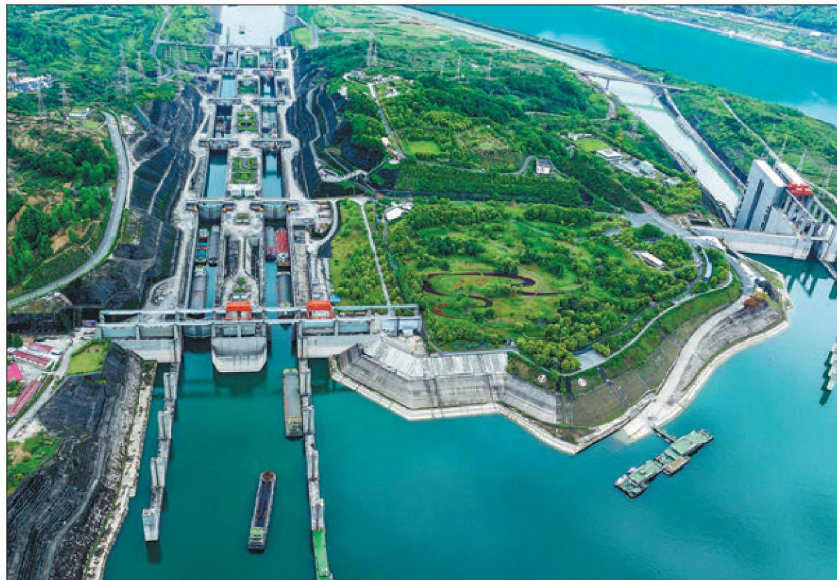
Ships pass through a lock on the Three Gorges Dam in April. The dam's annual freight volume has surpassed 100 million metric tons for the past five years. ZHENG JIAYU / XINHUA
