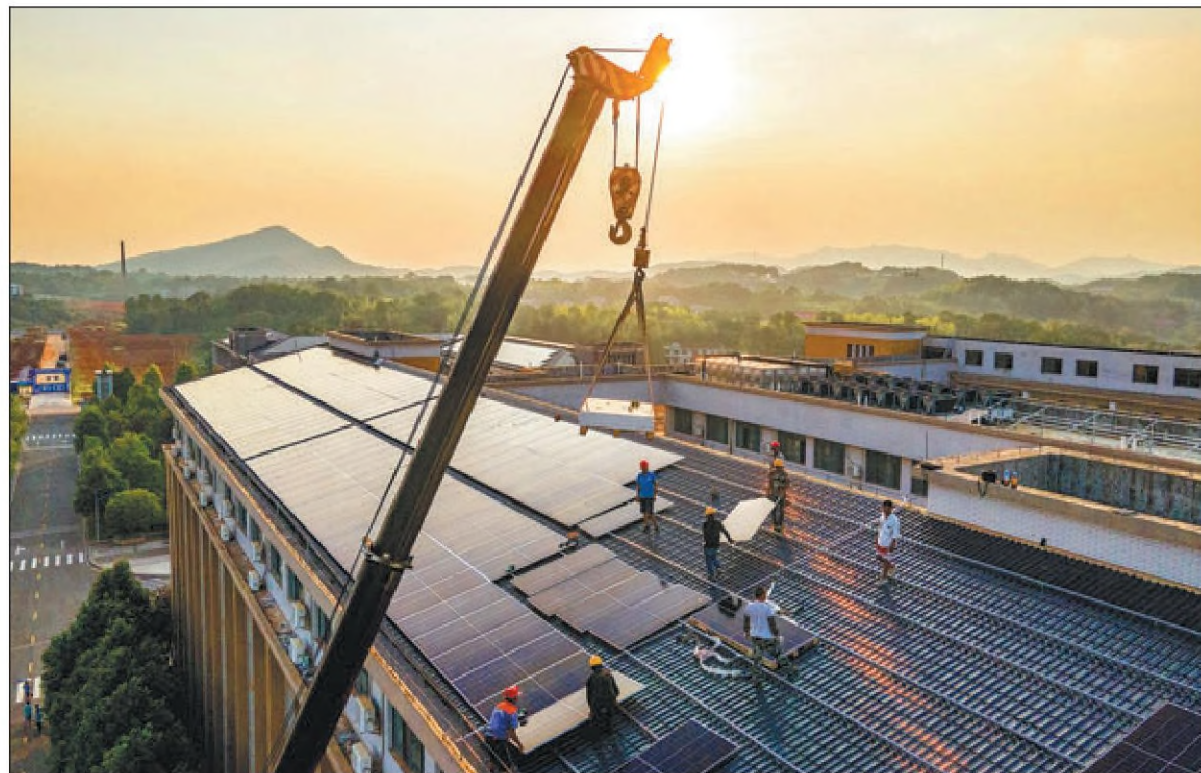
A crane is used to lift solar panels onto the roof of a building at the No 1 Middle School in Shuangfeng county, Hunan province, on Aug 18. PROVIDED TO CHINA DAILY
