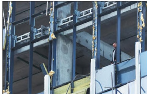
A security services member checks a damaged building following a reported drone attack in Moscow on Monday. MAXIM SHEMETOV / REUTERS
