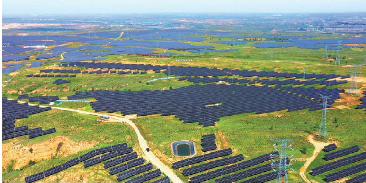
An aerial photo of the vast array of solar panels built as part of Tianjiao Green Power, a rehabilitation project aimed at balancing the environmental and economic development of coal mines in Ordos, Inner Mongolia autonomous region. PROVIDED TO CHINA DAILY
