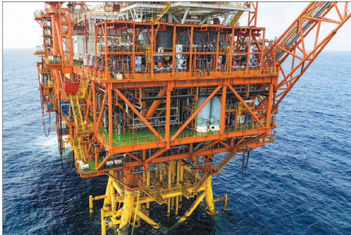
China's first offshore million-ton carbon storage project is put into operation on Thursday in the South China Sea. The project, serving the Enping 15-1 oil platform 200 kilometers southwest of Shenzhen, Guangdong province, is designed to capture and store more than 1.5 million metric tons of carbon dioxide, which is equivalent to planting nearly 14 million trees, according to the China National Offshore Oil Corporation.
