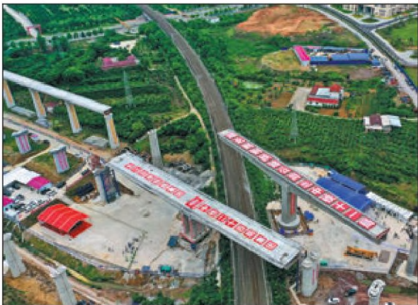
Two continuous T-beam bridges are rotated over the Jiaozuo-Liuzhou Railway in Jingmen, Hubei province, last week. The project is an undertaking partly built by China Railway 24th Bureau Group Corp Ltd. PROVIDED TO CHINA DAILY
