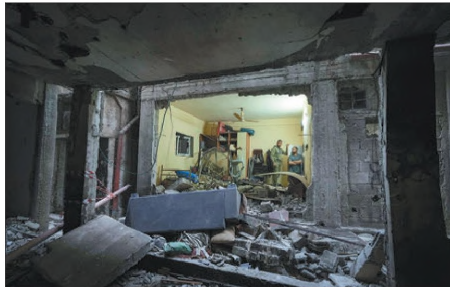
Palestinians inspect a damaged building following an Israeli army raid in the Balata refugee camp near the West Bank town of Nablus on Monday. Palestinian health officials say Israeli fire has killed at least three people in the refugee camp. MAJDI MOHAMMED / ASSOCIATED PRESS
