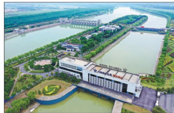
A pumping station on the eastern route of the South-to-North Water Diversion Project in Sihong, Jiangsu province on Friday. FANG DONGXU / FOR CHINA DAILY
