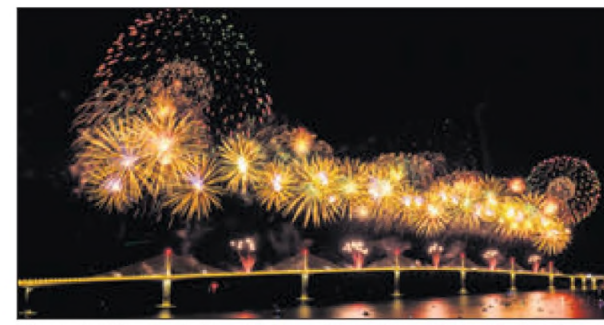
Fireworks illuminate the night over the Peljesac Bridge during its opening ceremony in Komarna on July 26. MIROSLAV LELAS / PIXSELL
