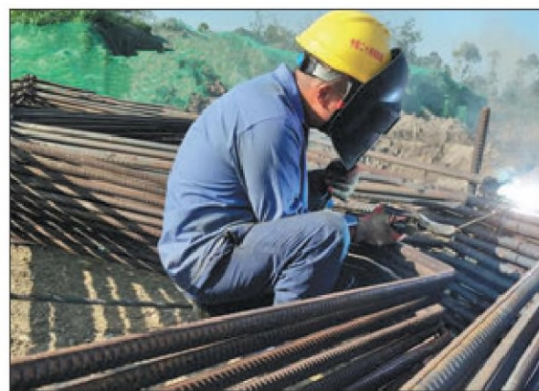
An employee of China Railway 24th Bureau Group Corp Ltd works on the Tianfu Avenue's northward road extension project in Deyang, Sichuan province. PROVIDED TO CHINA DAILY
