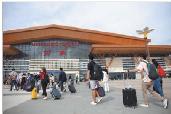
Travelers enter the railway station in Vientiane, Laos, to take the China-Laos Railway on Nov 25. KAIKEO SAIYASANE / XINHUA
