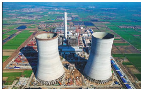
A thermal power station is under construction in Xiayang, Hubei province. ZHENG XINTAO / FOR CHINA DAILY
