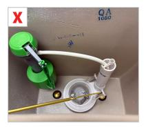
Do NOT insert the refill tube below the water level inside the overflow tube, as this can cause the tank to slowly siphon into the bowl.
