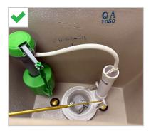
This positioning ensures an air gap between the refill tube outlet and tank water level, which is required to prevent siphoning.
