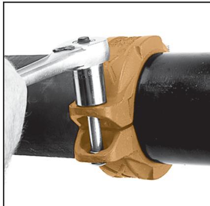
**5 TIGHTEN NUTS—** Securely tighten nuts alternately and equally to the specified bolt torque, keeping the gaps at the bolt pads evenly spaced.
