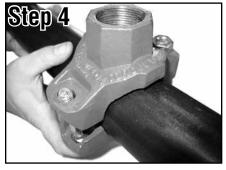
Alignment Align the strap around the pipe, insert the bolts and tighten the nuts finger tight.
