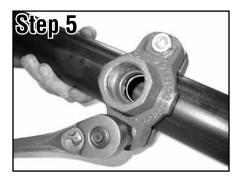
Tighten nuts Alternately and evenly tighten the nuts to the specified bolt torque.
