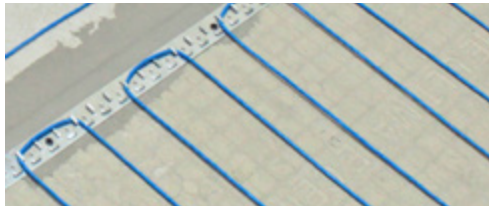
WarmWire installed using CableStrap
