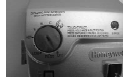
Gas Control shown in the "OFF" position
