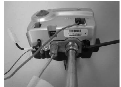
Gas Control shown in the "OFF" position
