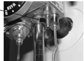
Pressure Tap Shown Installed
