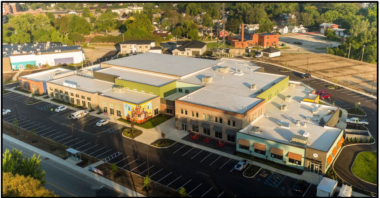
An aerial view of Northend Community Center
