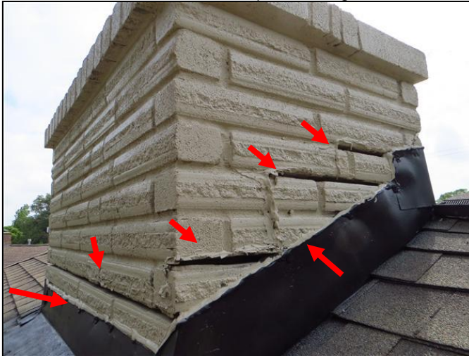
Through-wall metal counter flashing embedded in masonry.
