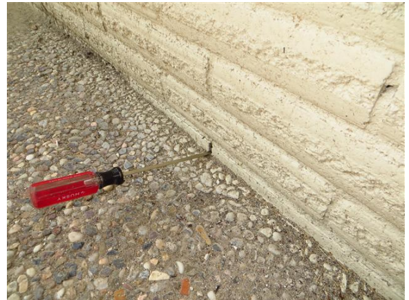
Weep holes - vented rain screen principle
