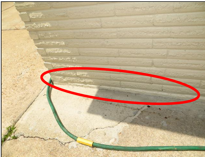
Weep holes - vented rain screen principle
