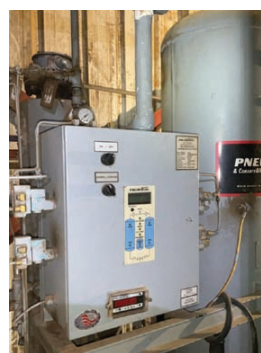
Pneumatic Air Dryer Model PE-650, SN: 0106-S135899-025763, 7.5 kw heater, 460V 3 phase, 650SCFM, Desiccant air dryer, no pipe past line filters, working unit.
