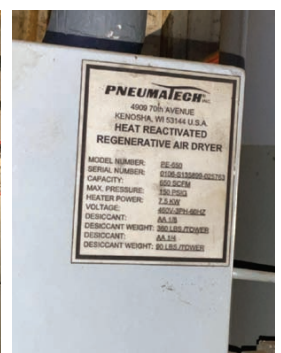
Pneumatic Air Dryer Model PE-650, SN: 0106-S135899-025763, 7.5 kw heater, 460V 3 phase, 650SCFM, Desiccant air dryer, no pipe past line filters, working unit.
