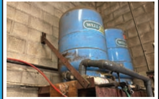
Well Trol Pressure Bladder Tank 50 Gal — Description — Model WX-302 max pressure 100PSI
