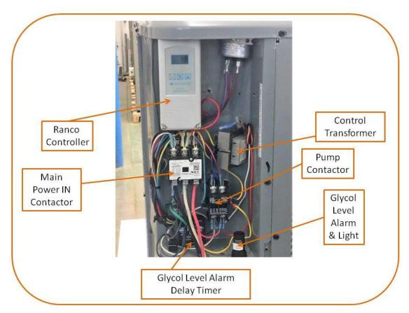
There is a 24V Controller transformer in the cabinet. On the primary side, it has an orange wire for 230/240 volt power, or a red wire for 208/220 volt power (see label on transformer). You will see one of those 2 wires at the transformer will be capped. Depending on what voltage your facility has, you can swap the red for the orange, or vice versa to
