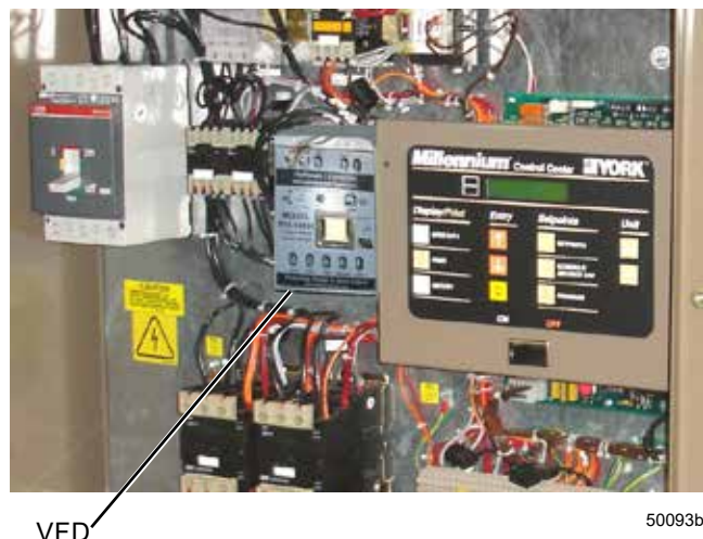
FIGURE 45 - TYPICAL VFD LOCATION
