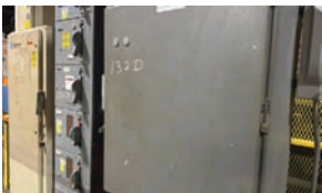
Motor Control Center For Edger
