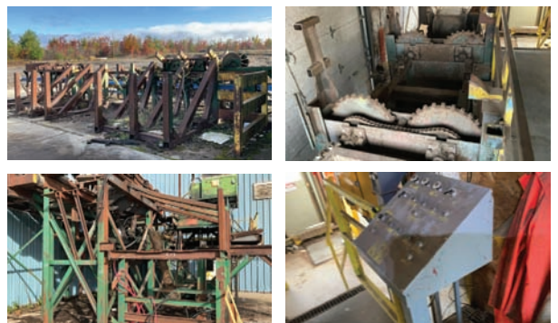
Steel sub structure
