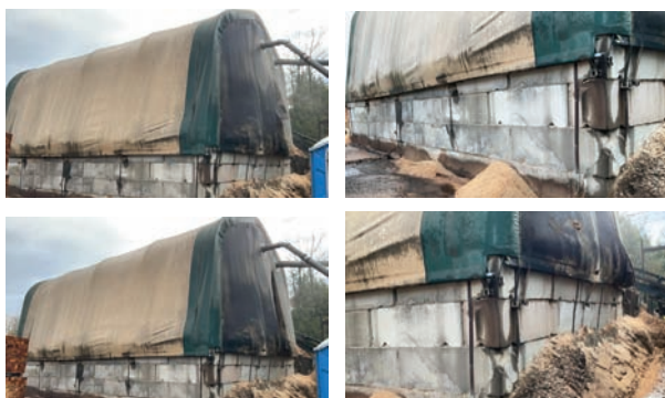
Hoop Building — Description — 30' x 48' Tube truss frame.
