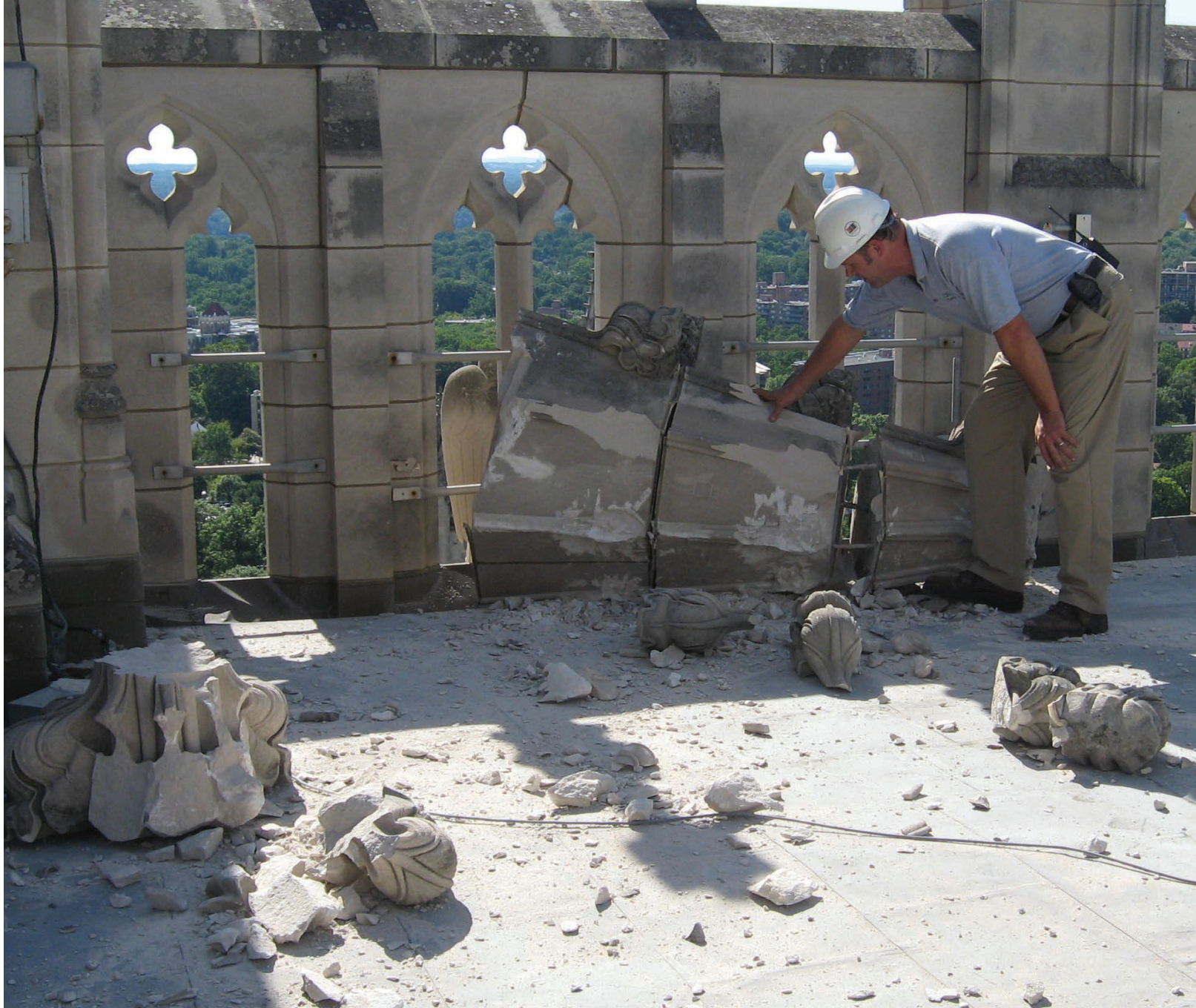
For forty years head mason Joe Alonso has tended to the stone needs of the cathedral. Here he begins "mason triage" during early visual assessments after the rare 5.8 magnitude earthquake shook the 118-year-old structure to its core. Image courtesy of Washington National Cathedral
