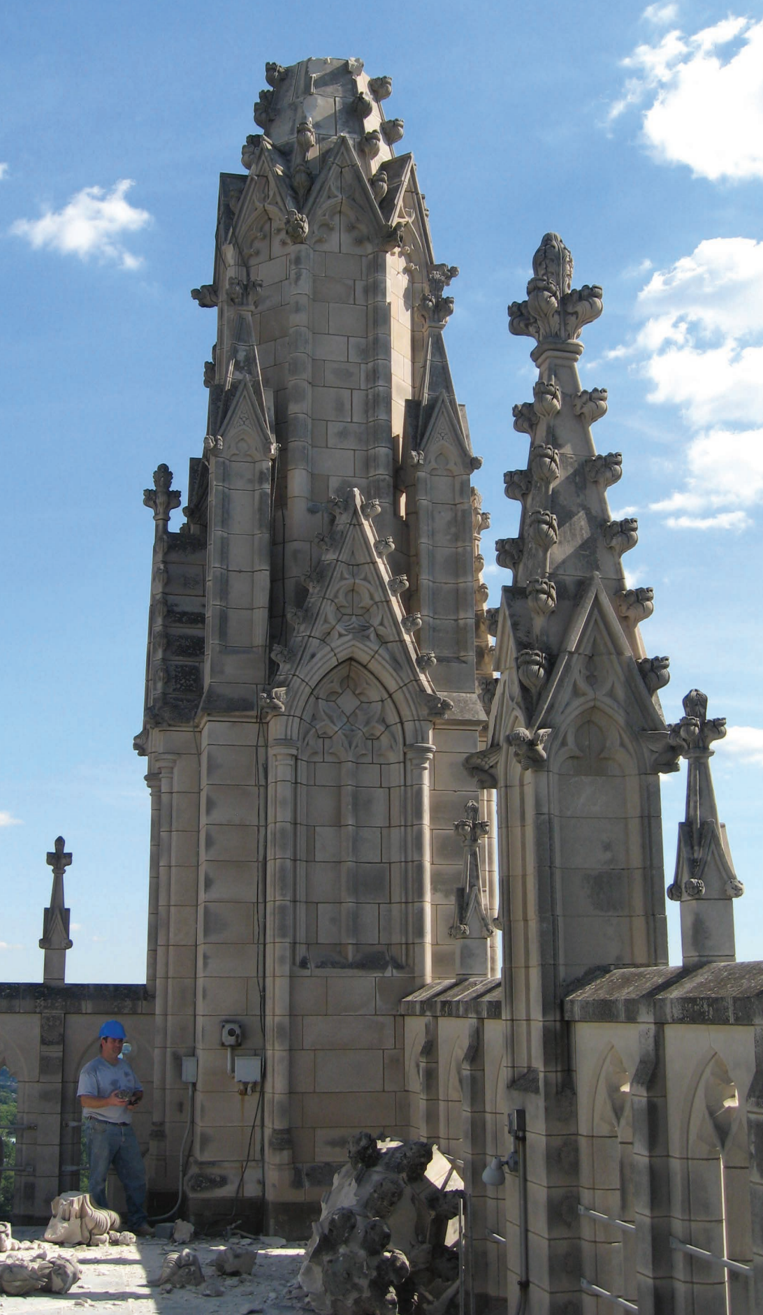
More than 75% of the cathedral’s pinnacles were damaged, including all four grand pinnacles. Image courtesy of Washington National Cathedral
