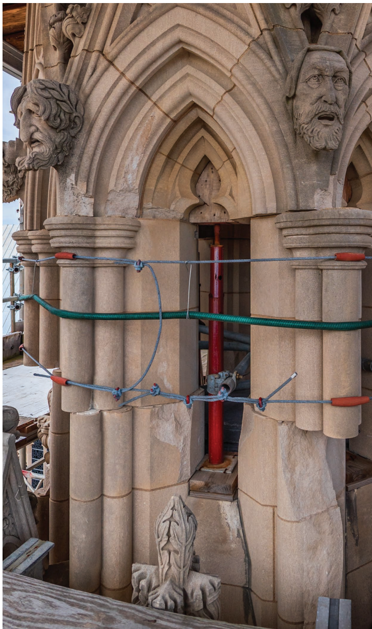
Above and opposite page before and after images. The earthquake shook the elements of the cathedral, loosening the stones. This is one of the grand pinnacles of the south transept, which rotated severely on eight slender columns that supported almost 30 tons of limestone. The pinnacles were disassembled, structurally enhanced and reassembled. Photo courtesy of Lorton Stone, LLC
