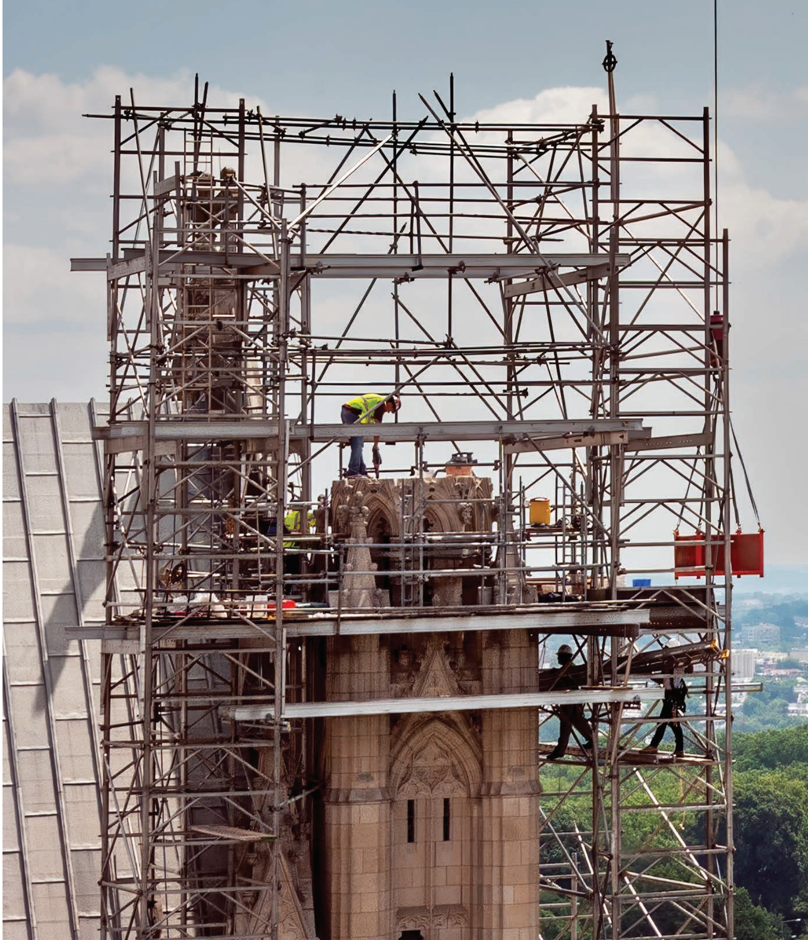
Painstaking work takes place high above the city. Building the scaffolding alone can take months. Then damaged or unstable stones are removed with a crane. Salvageable stones are taken into the shop to be repaired, and if needed, new pieces are made. Then structural upgrades are completed and the stones re-set with a crane. Photo courtesy Lorton Stone, LLC
