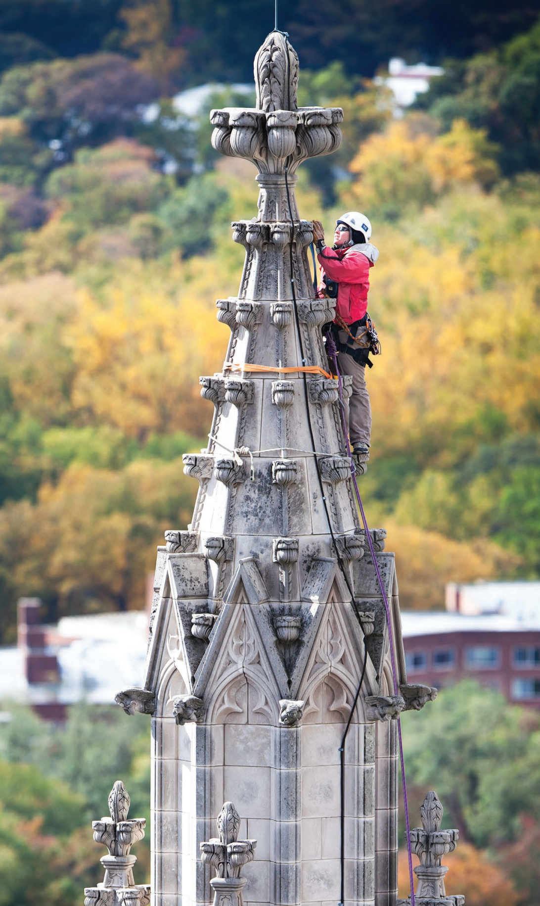
The rope access team from Wiss, Janney, Elstner Associates rappelled off the exterior to inspect stone and continue the 'pick and clean' process to remove loose and unstable material that otherwise might remain and potentially become disrupted downstream. After this point, the team felt confident that the public could safely return. Photo courtesy of Wiss, Janney, Elstner Associates
