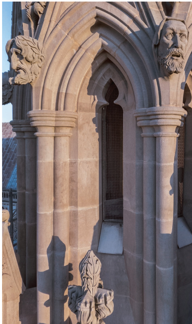
Above and opposite page before and after images. The earthquake shook the elements of the cathedral, loosening the stones. This is one of the grand pinnacles of the south transept, which rotated severely on eight slender columns that supported almost 30 tons of limestone. The pinnacles were disassembled, structurally enhanced and reassembled. Photo courtesy of Lorton Stone, LLC
