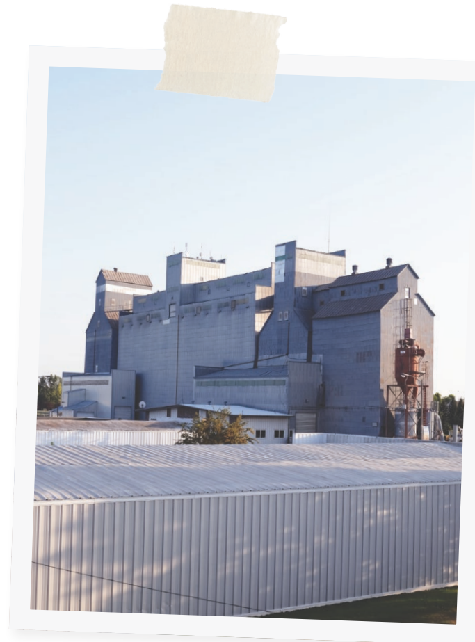
Hallock Co-Op Elevator Co.
