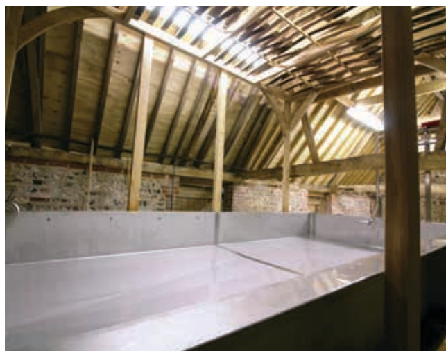
Burning Sky's coolship carefully installed in the rafters above the barrel store
