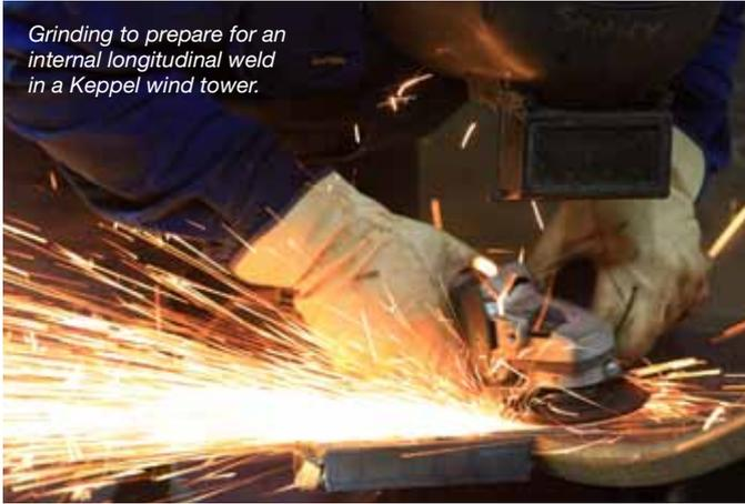
*Back grinding to prepare for internal submerged arc welding.*
