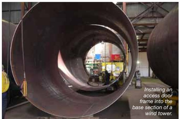
*Installing an access door frame into the base section of a wind tower.*
