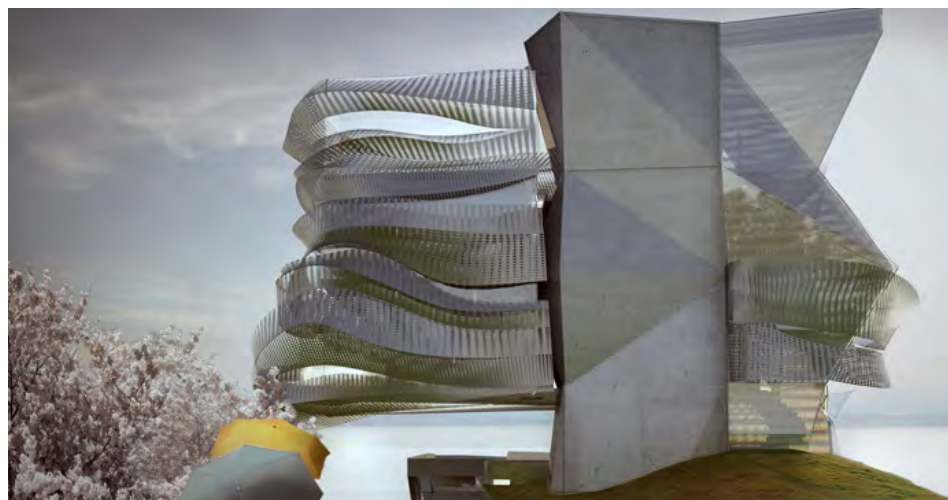
A rendering of the “House of a 1,000 Views” (unbuilt), designed by Do[Su Studio Architecture, shows an integration of smart and passive solar shading systems. Photo courtesy of Do[Su Studio Architec-
