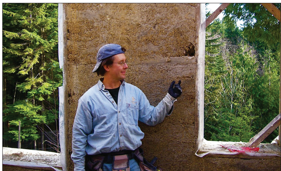
At left: Hempcrete CEO Kim Brooks isn't afraid to get hands on and apply a deep coral wall colour crafted with pigments from the earth. At right: Jayeson Hendyrsan stands in front of a rough wall. The pre-plastering stage shows the industrial hemp fiber used in the lightweight fiber reinforced concrete. photos supplied by Hempcrete.ca
