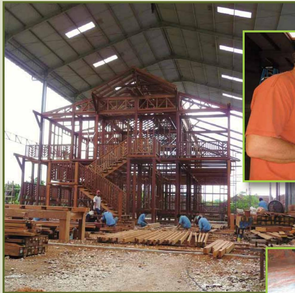
Pictured above, the custom-designed home was pre-assembled in Bali, then disassembled and shipped to Kona in containers. The Teak Bali company worked directly with the Buckingham's and their locally based architect, Neil Erickson, of Hilo.
