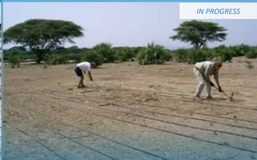
This photo shows a particular area "before" and "after" the installation of the community gardens.
