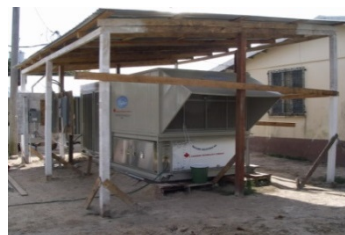
Figure 2: 2500 L/day water-from-air system (mechanical dehumidifier; commercial product) in Belize City. Photo by author.
