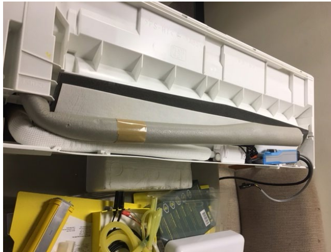
The above image shows the X85-003 hidden behind the unit. If hidden behind the unit, the refrigerant piping will not be able to be run in the same area as the pump.
