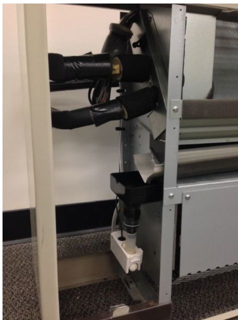
Example of PFFY condensate reservoir installation
