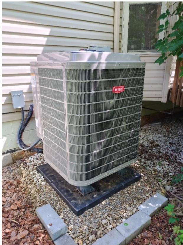
Figure 5. Bryant model 284ANV048 outdoor unit.
