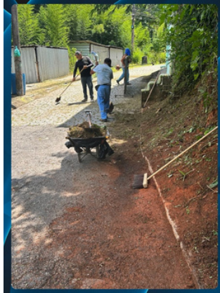
ROÇADA E LIMPEZA Rua Afonso Sardou, Village
