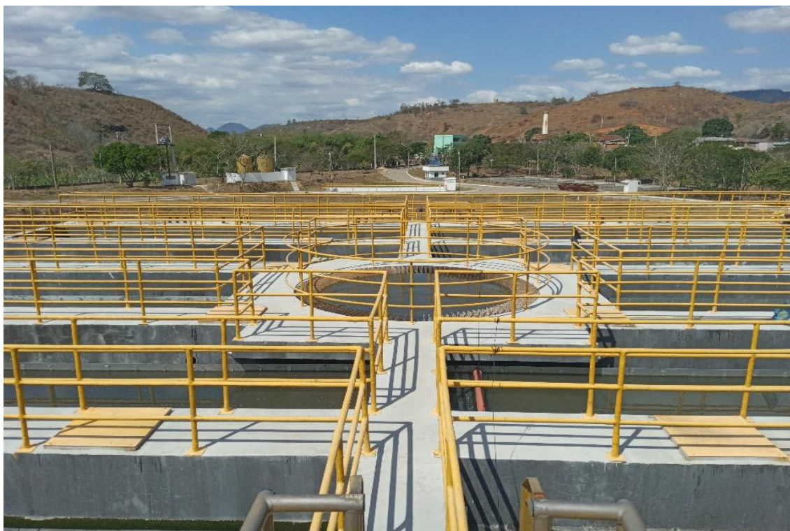
Figura 03: Reator UASB
