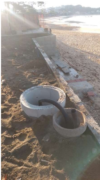
VALA REATERRADA MANUAL
