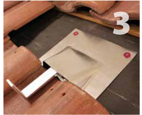
Install the sub-flashing over the base and hook. Fasten the sub-flashing into place with two roofing nails, one in each top corner. Clean away dust and debris.
