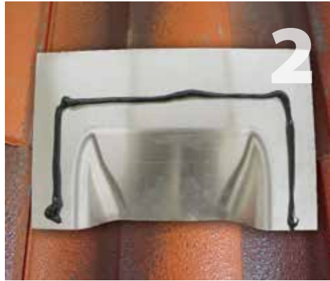
Apply a bead of sealant in the shape of an upside down U on the back side of the sub-flashing.
