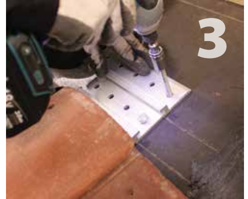
3 Connect hook to base plate and drive lag screws into rafter through the two holes to a solid, snug fit. DO NOT over tighten lag screws, this may compromise their holding strength.
