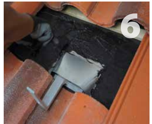
After first layer of cement is dry, apply second layer over reinforcing fabric to finish waterproofing of sub-flashing.
