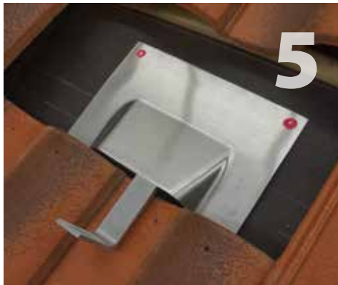
5 Carefully clean the underlayment then apply bead of sealant compatible with roofing materials in the shape of an upside down U on the backside of the sub-flashing, see example on page 2, and install flashing over mount. Fasten sub-flashing to deck with one roofing nail in each top corner. Do not nail bottom corners.
