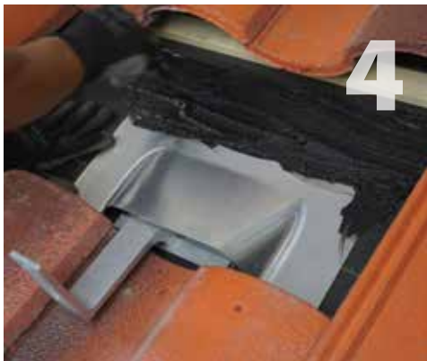
Apply 1/8" thick layer of roofing cement around the top and sides of the sub-flashing with at least 1" extending past the sides of the flashing onto the felt.
