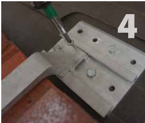
4 Slide hook into desired position within valley of the tile. The hook must not overhang the side edges of the base plate. Drive self-tapping screw to secure hook to base using a #3 Phillips drive bit. Do not use impact gun on screw.
