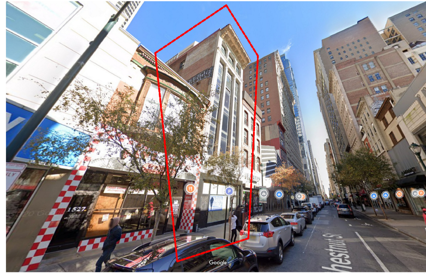
4 VIEW EAST ON CHESTNUT STREET Z2
