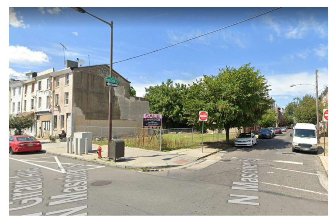
2 VIEW AT CORNER OF W GIRARD AVE AND MASCHER ST SP-2 N.T.S.
