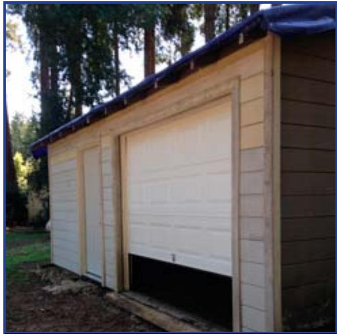
Pool house garage, the whole back wall was replaced, and the concrete footing was extended all the way across the back, under these two new doors. Termites and dry rot ate away all the posts and framing holding the whole back wall together.
