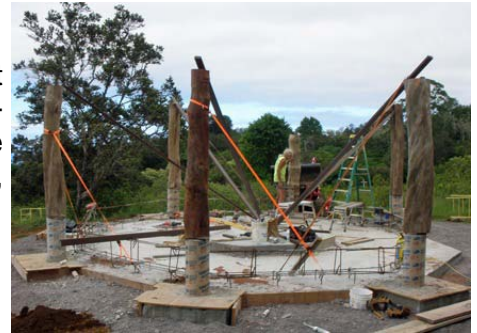
Ohia logs supporting the chapel structure.
