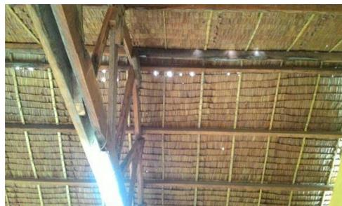
The roof of the church building is temporary made of palm leaves. And needs to be replaced
